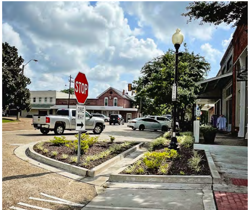
See how a downtown community used strategic design in their bulbout to address stormwater drainage.
