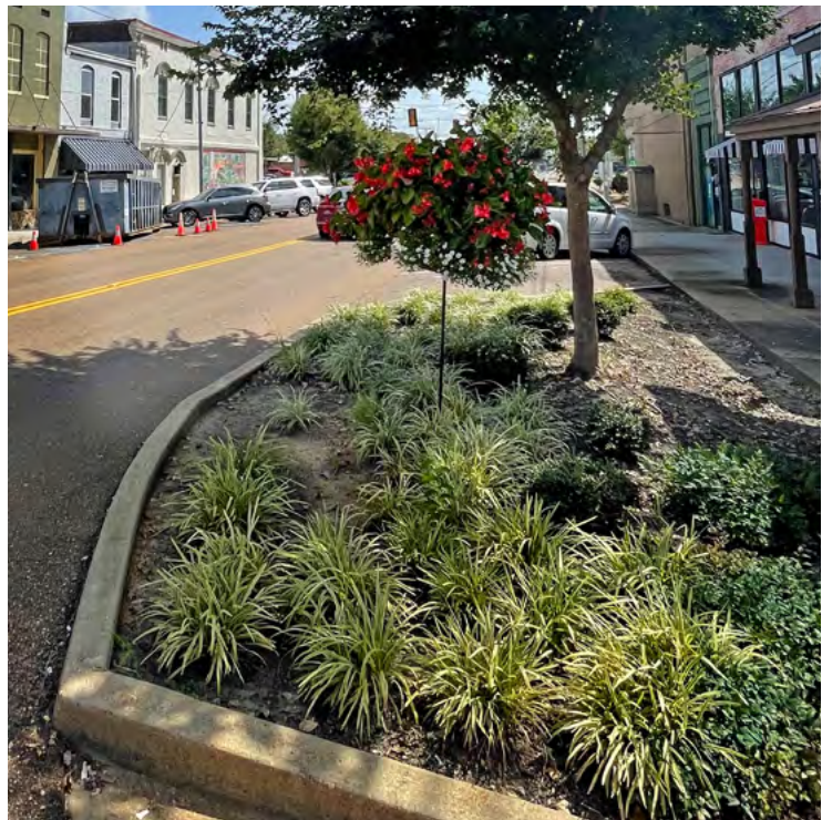
Bulbouts are also an opportunity to introduce street trees into your downtown. Bulbouts provide ample space for your trees to grow and in return, the trees offer shade and cooling effects for your downtown.
